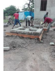
construction of tank base
