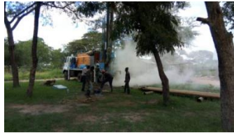
Machine starting drilling
