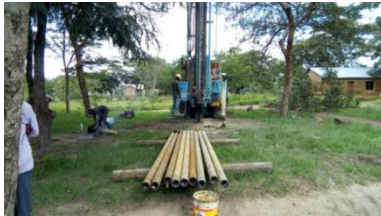
Machine for borehole at site
